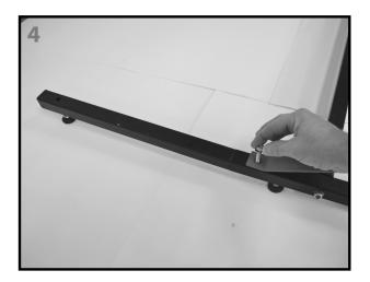
. Firmly tighten 50mm bolts using 1/2" wrenches. See image 5.
